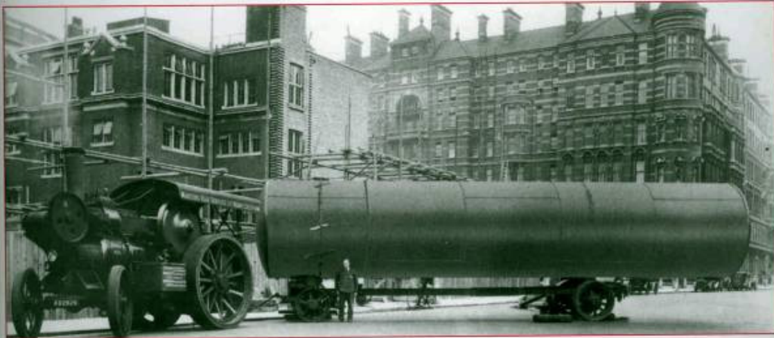
1930 Imperial College of Science, London (Delivery of a large hot water calorifier by Sulzer Bros)
