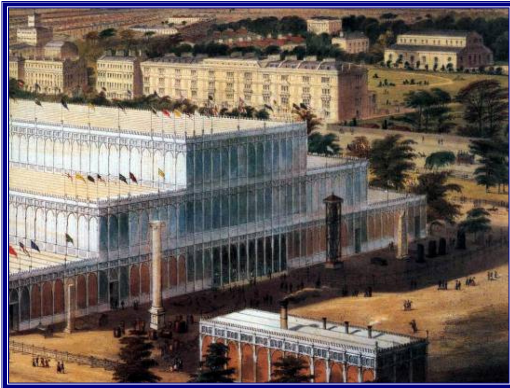
Detail of the Crystal Palace in Hyde Park; the boilerhouse (bottom centre) produced steam to drive exhibits in the Machinery Hall; the building was unheated
