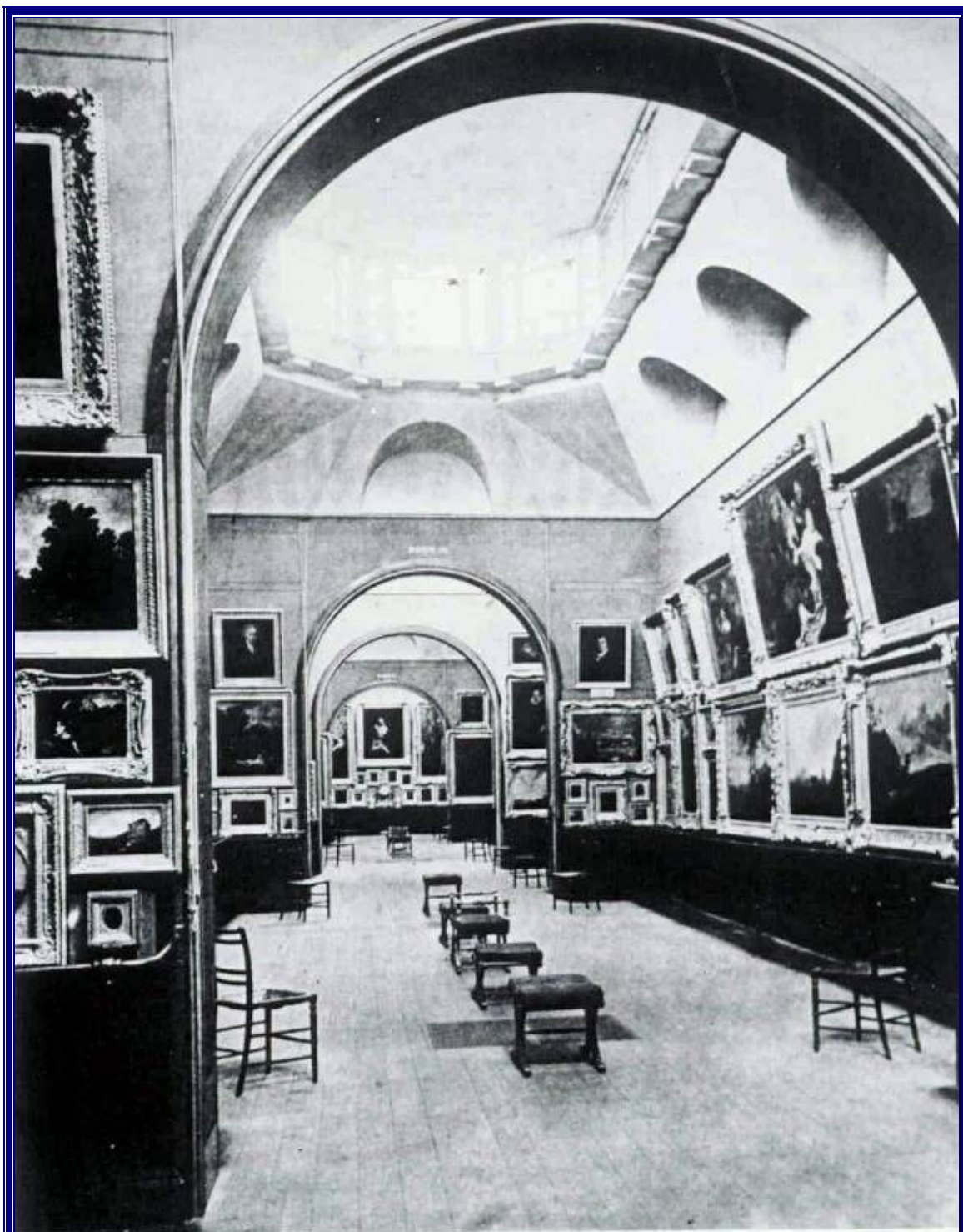
19 Vista through the gallery at Dulwich. Photograph taken c. 1900, still with the original glazing of Soane's lantern.
