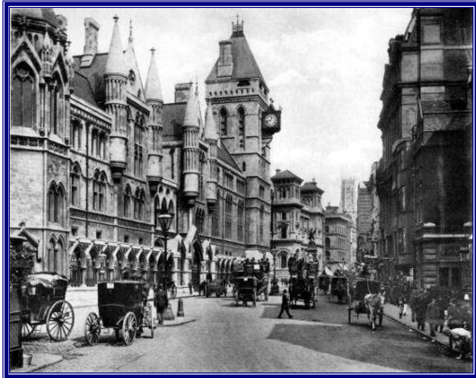
The Royal Courts of Justice in the Strand (an early photograph)
