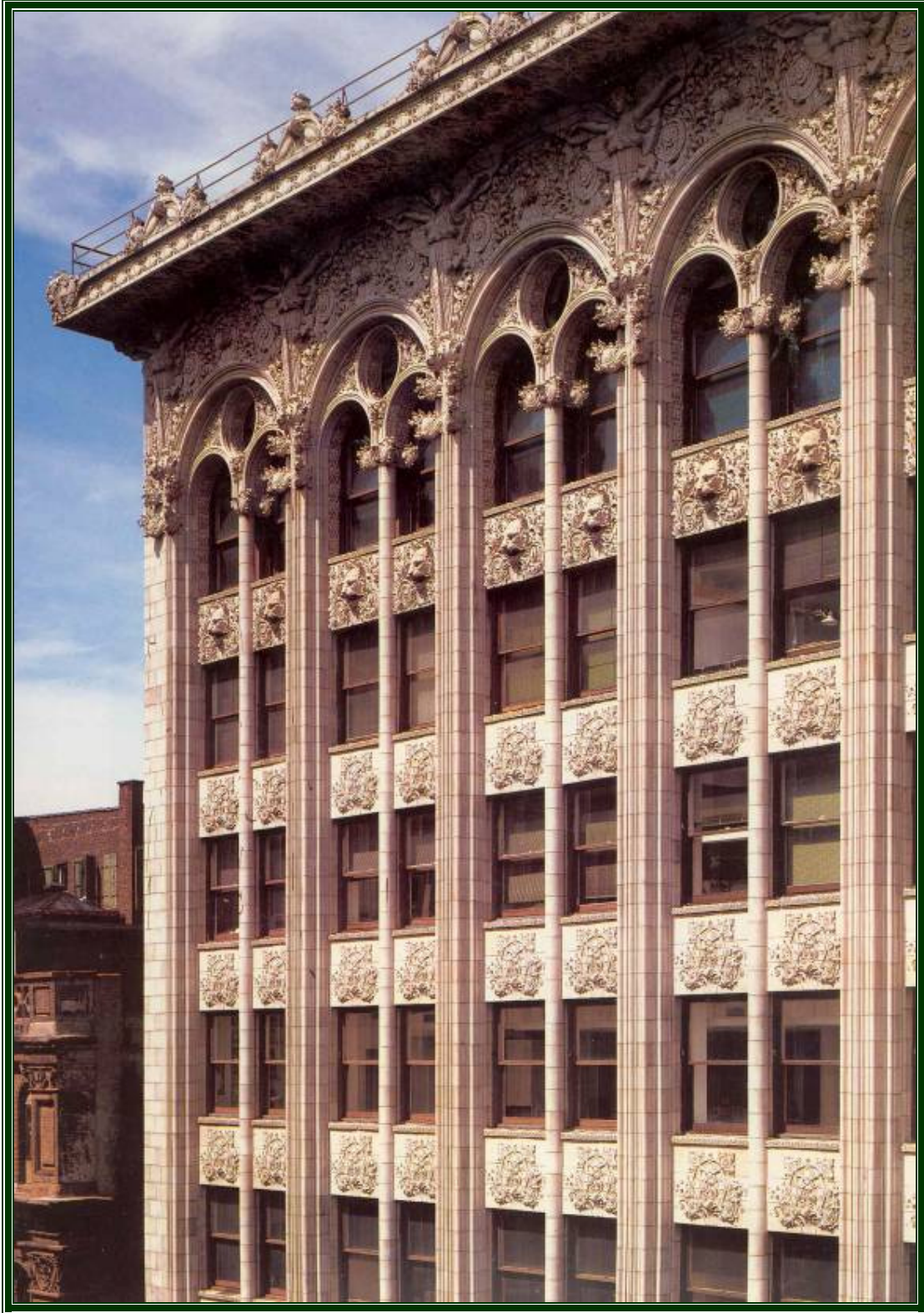
Bayard Building, New York City, 1897
