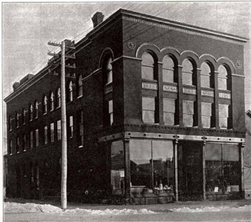
PLUMBING, GAS, STEAMFITTING AND BICYCLE STORE OF JAMES A. TRANE, LA CROSSE, WIS.
