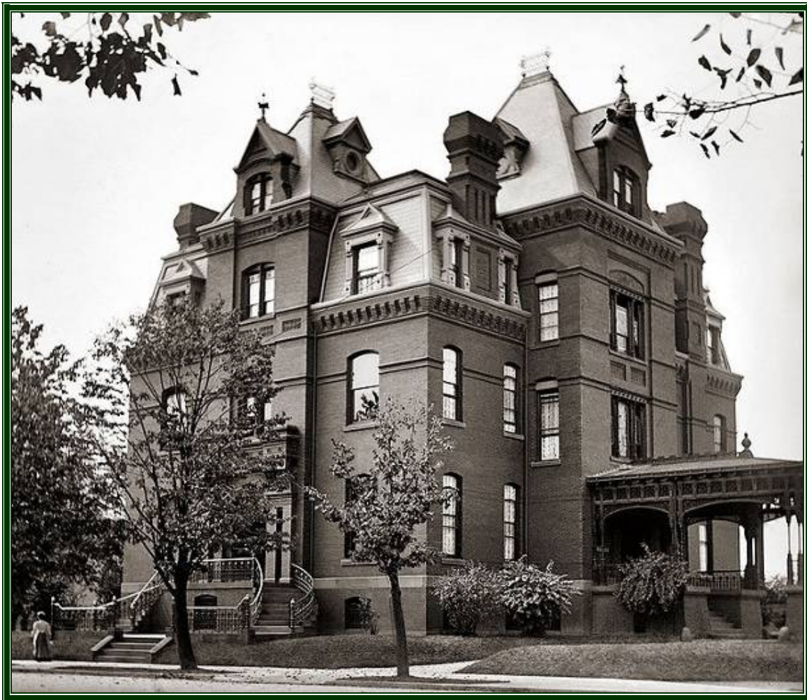
Blaine Mansion, Washington DC: Home of Westinghouse
