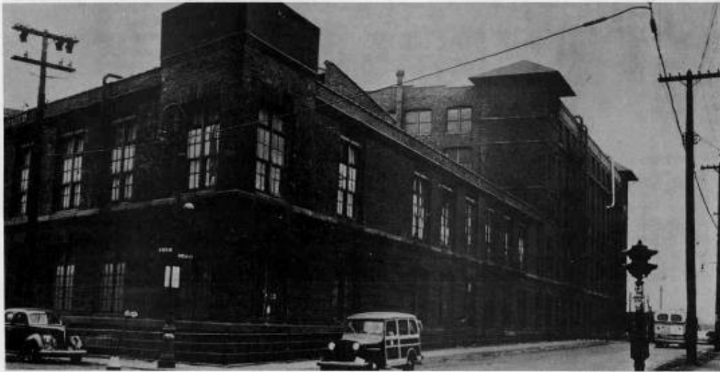
Fig. 1 The first scientifically engineered air-conditioning system was installed in 1902 in the Sackett-Wilhelms lithographing and printing plant in Brooklyn, N.Y.
